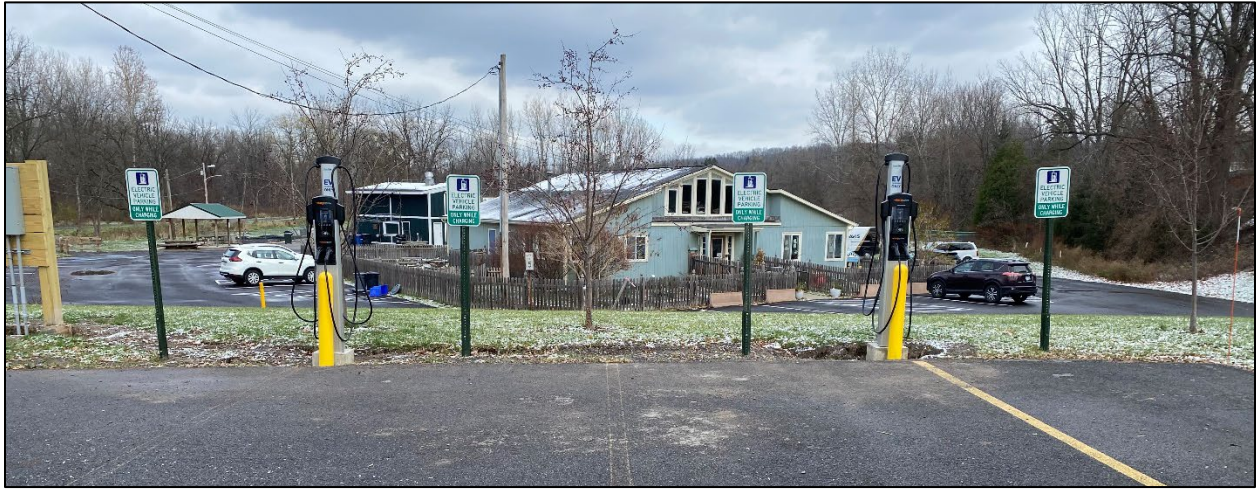
Figure 6: Mostly funded by state and utility grants, in November 2022, the Town installed two dual port level 2 EV charging stations at Town Hall that are available to the public.
